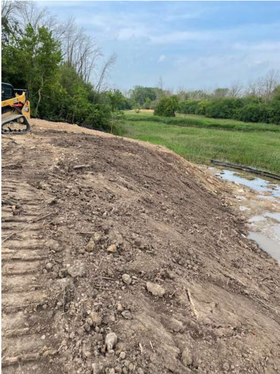
Excavated slope of the flood storage area.
