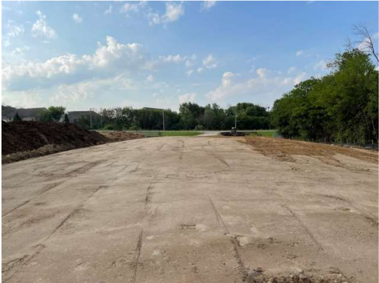
Applied borrow material on the southern end of the project.
