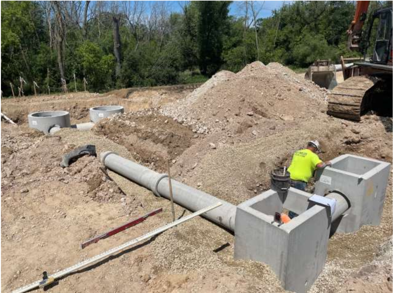
Storm sewer structure installation on the north end of the project.
