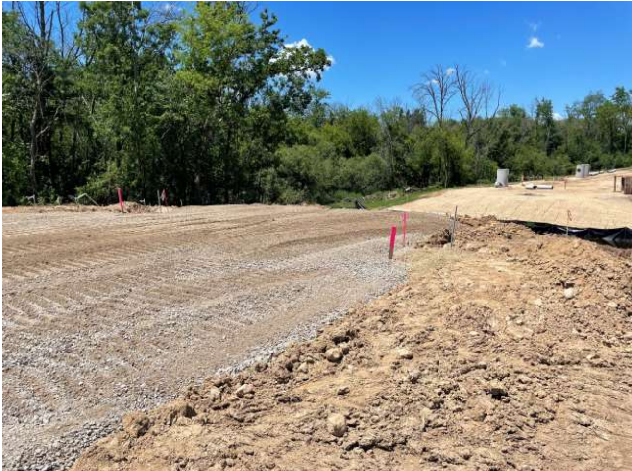
Base layer before compaction on the south side of the project.
