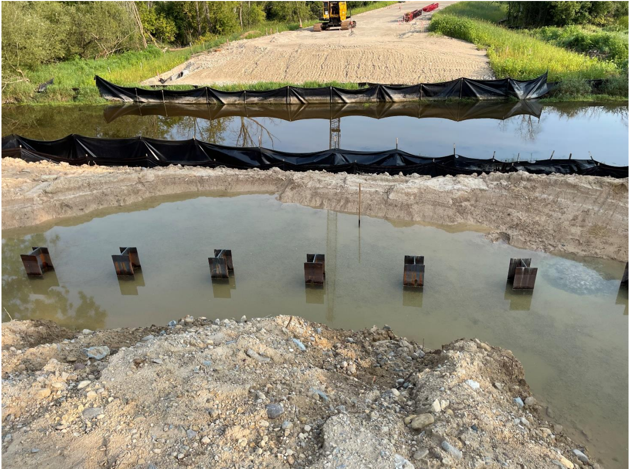
Driven piles on southern abutment post rainfall.
