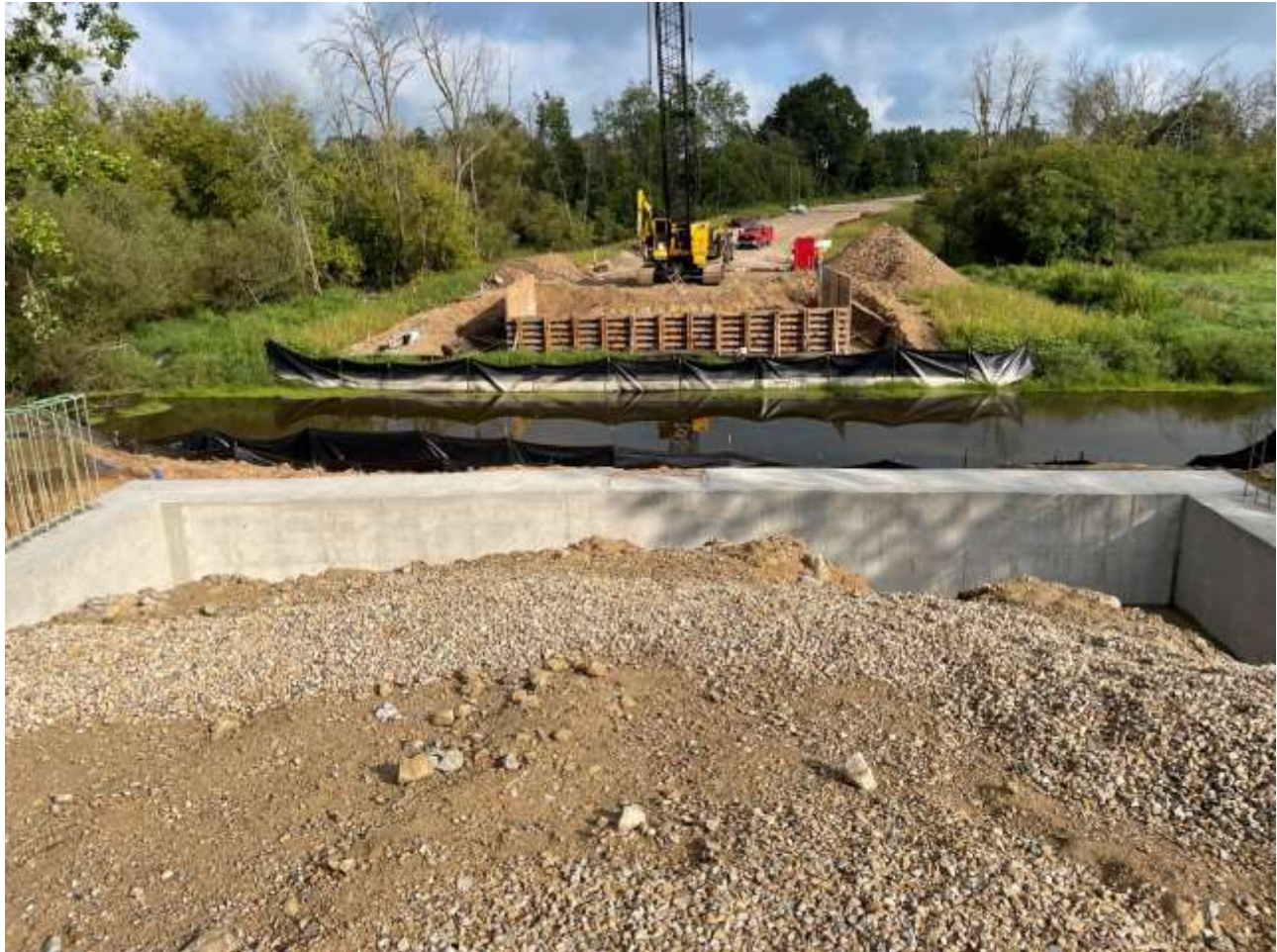
Southern abutment structure with view of northern abutment formwork.
