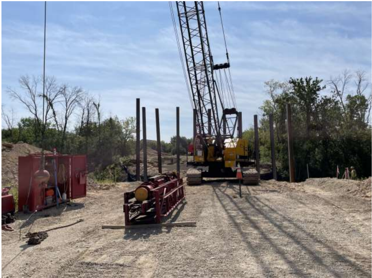
Driven piles for the northern bridge abutment, before cutting to size.
