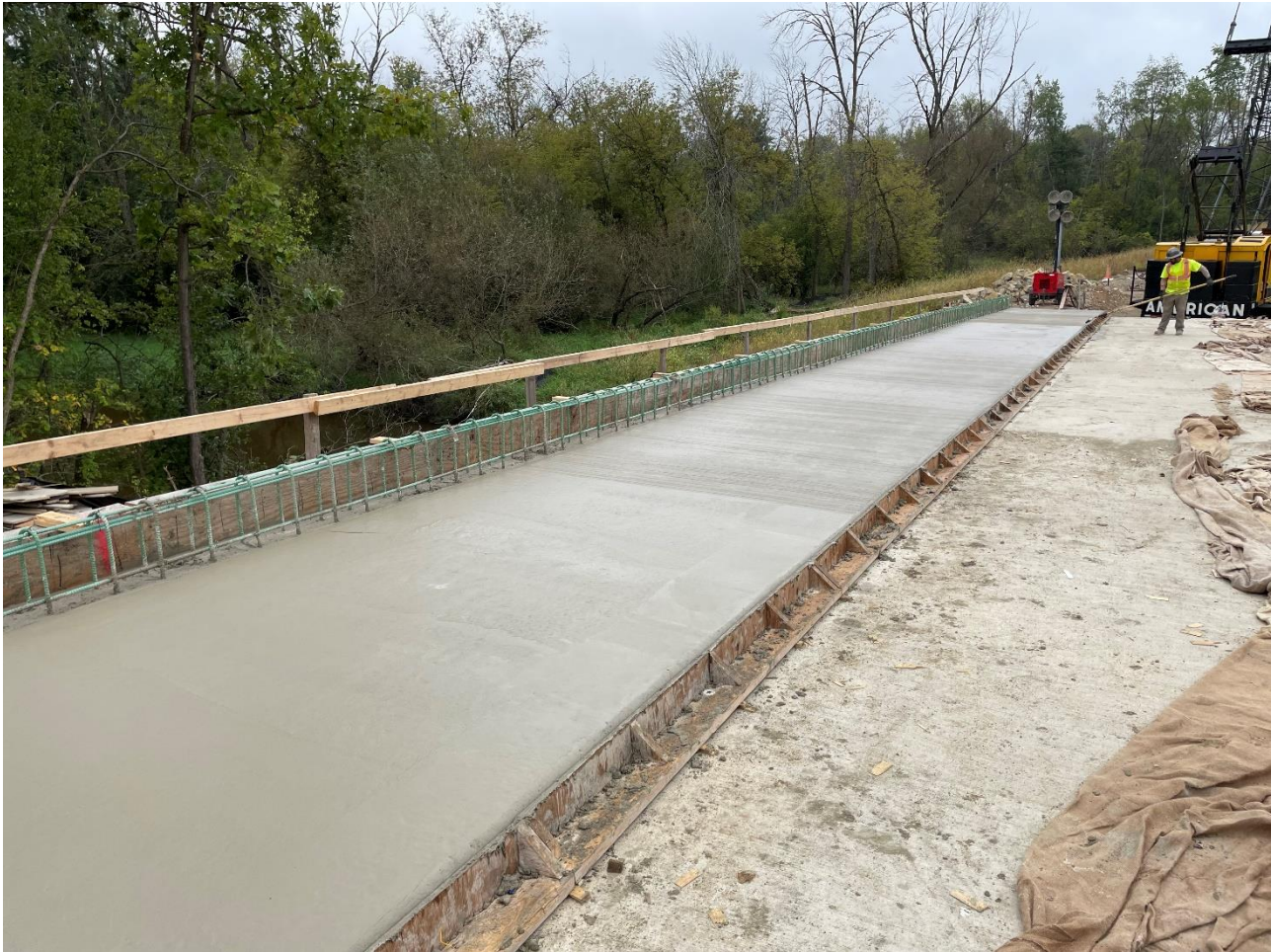
Western bridge sidewalk after pouring and before curing
