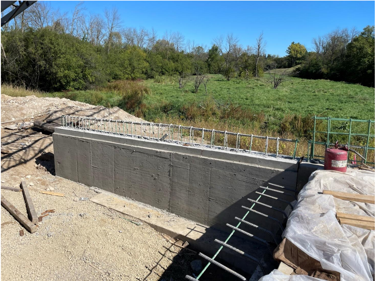
Top of Wingwall #4 after form removal
